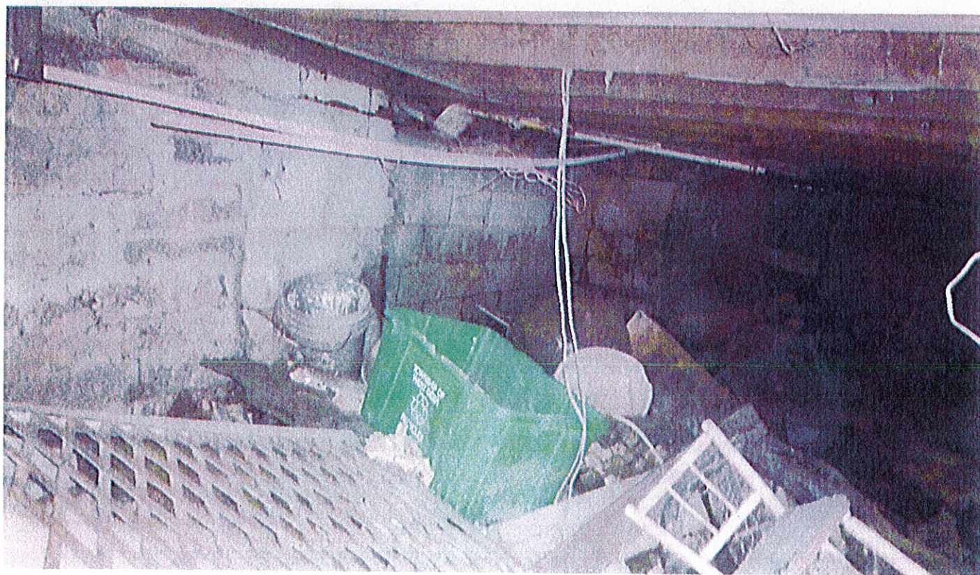
Basement from only access #3 side
